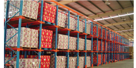
Drive Through Racking
